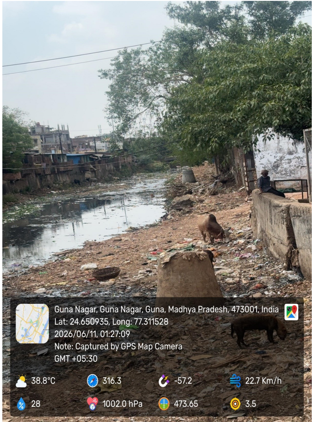
Figure 9: Pollution at Haat Road stretch
