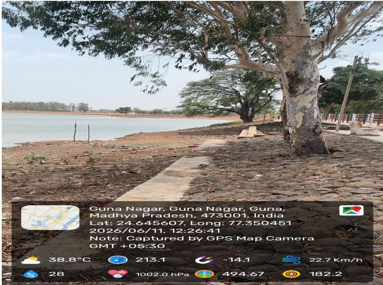
Figure 4: Existing riverfront work at Singhwasa Talab
